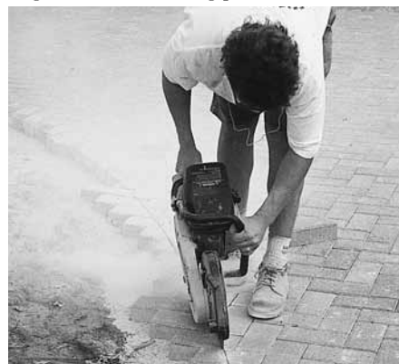
Figure 8. Saw cutting pavers.
