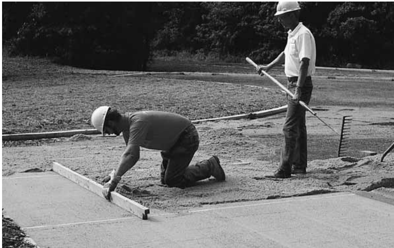
Figure 6. Screeding the bedding sand.
