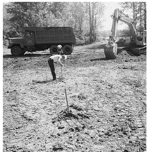
Figure 1. Excavation of the soil subgrade.
