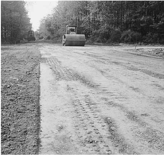
Figure 2. Compacting the soil subgrade.
