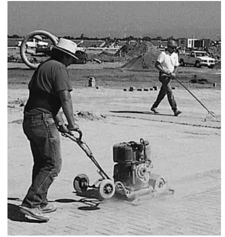
Figure 11. Vibrating sand into the joints.
