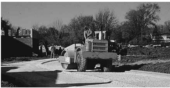
Figure 4. Base compaction with a vibratory roller.
