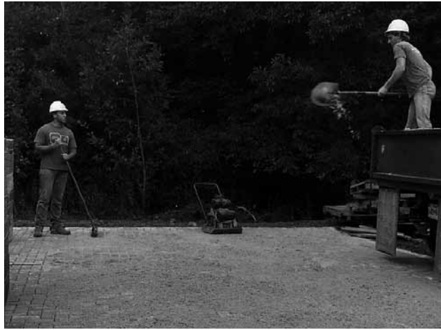
Figure 10. Spreading and sweeping joint sand.
