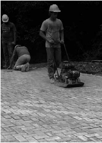
Figure 9. Compacting the pavers and bedding sand.
