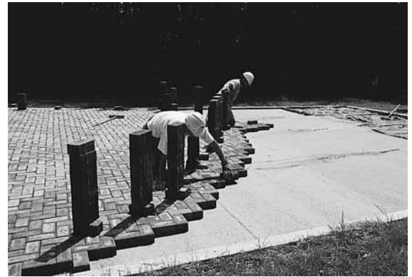
Figure 7. Placing the concrete pavers.
