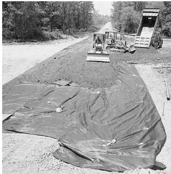
Figure 3. Application of the geotextile under aggregate base.
